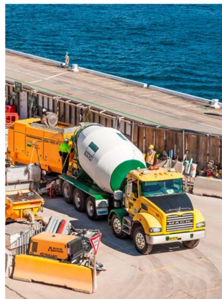
Delivering concrete to Barangaroo project
