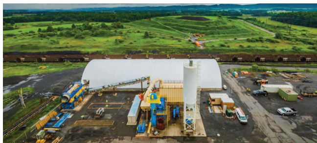
Boral North America's landfill reclaim operation at Montour, Pennsylvania
