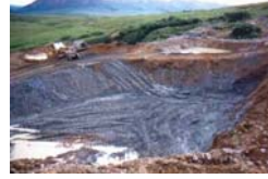
Site Services and Disposal
