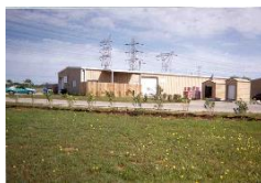
1,200 sq ft Bruanig Lab, adjacent to plant
