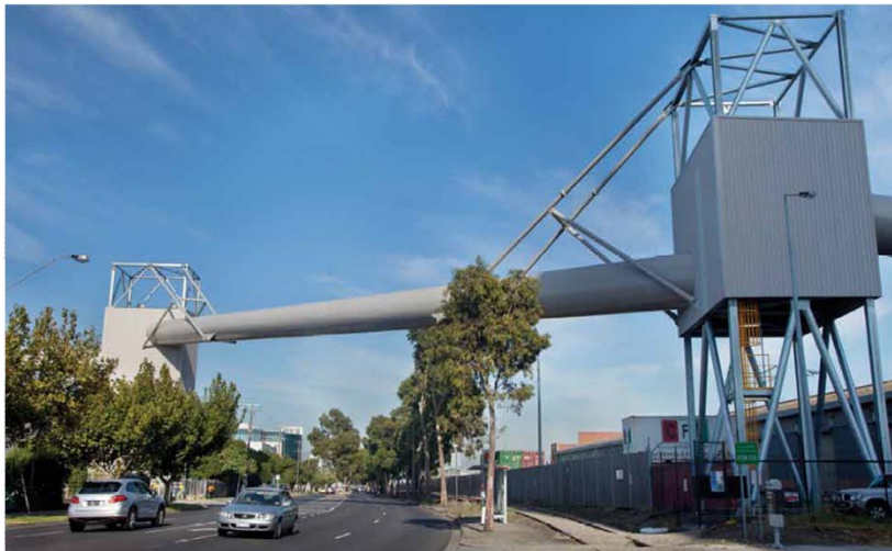
The new gypsum receiving/conveying system over Lorimer Street
