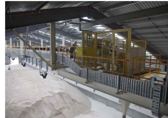
The new 40,000 tonnes gypsum store
